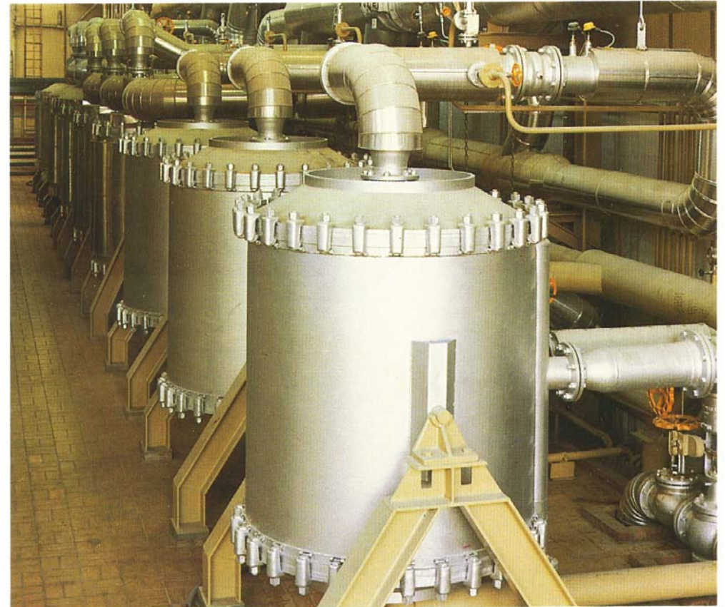
Seven Alfa-Laval spiral heat exchangers heat prelined sugar juice at Coop. Vereniging Suiker U A, Puttershoek, the Netherlands.
