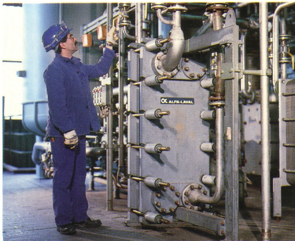
Hoechst AG in Frankfurt-Griesheim, West Germany, selected the Diabon F graphite plate heat exchanger for its excellent corrosion resistance when cooling a highly corrosive hydrochloric acid solution.
