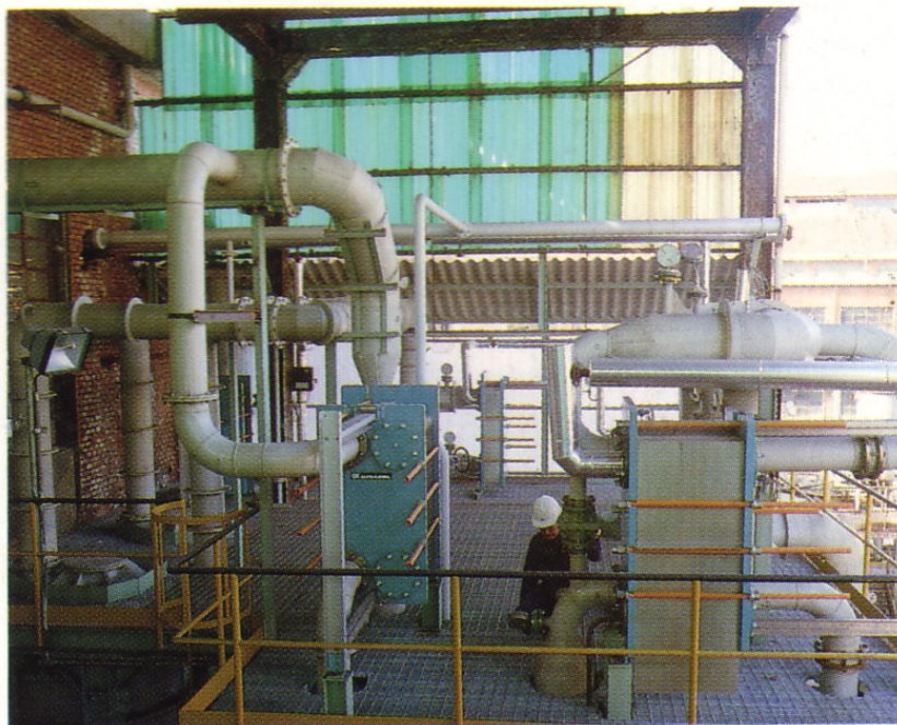
ACNA, a member of the Montedison Group, located in Cengio, Italy, chose four Flow-Flex plate heat exchangers for cooling contaminated air to remove dangerous chemical residues.
