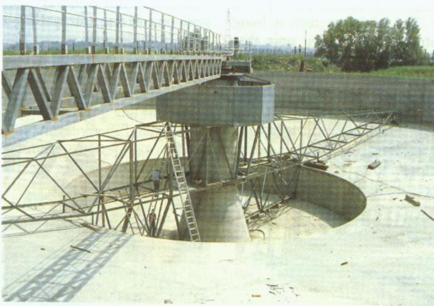
Figure 308. Valenton (Paris area, France) facility for SIAAP. Flow: 300,000 \text{ m}^3.\text{d}^{-1} . Central drive unit on the concrete centre column of a primary settling tank, 52 m dia.
