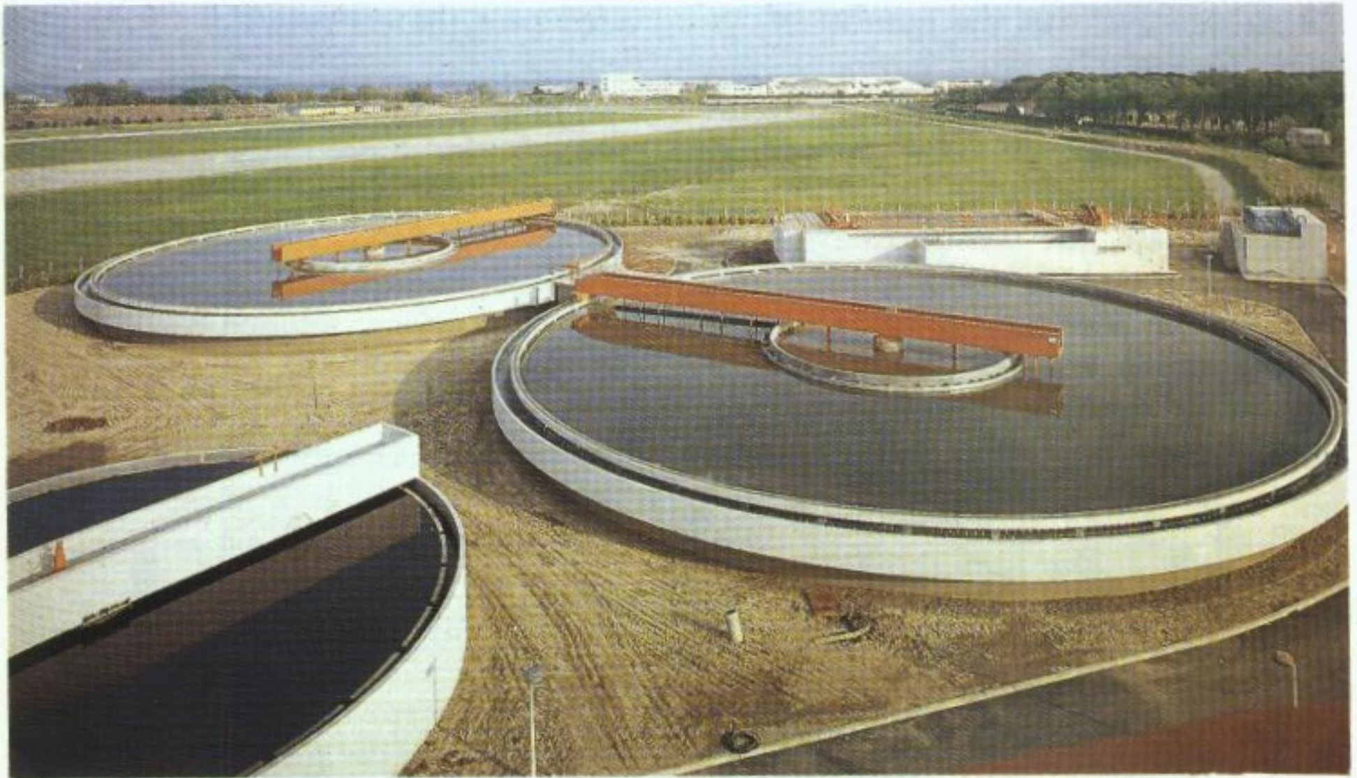
Figure 310. Cannes (Southern France) facility. Maximum flow: 5,500 \text{ m}^3 \cdot \text{h}^{-1} . Flocculator/settling tanks.
