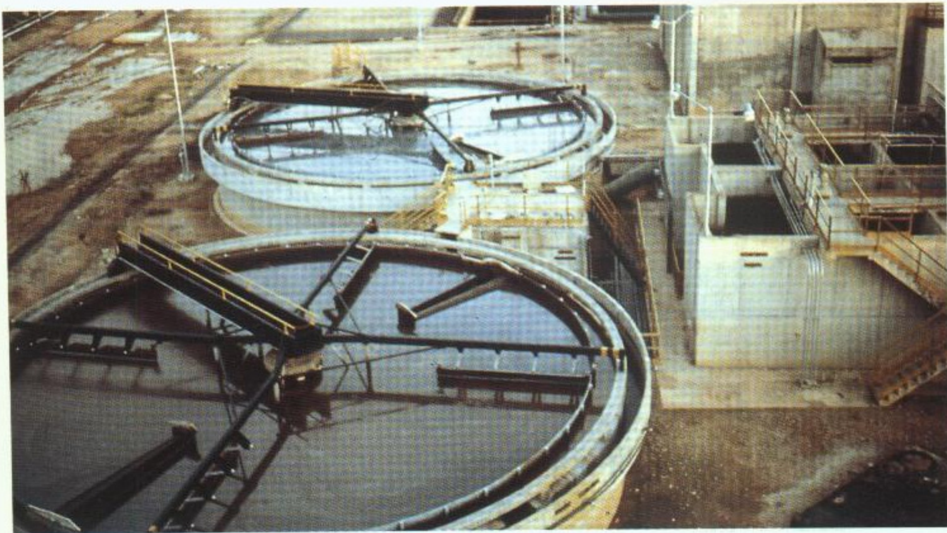
Figure 358. Barrancabermeja (Colombia) facility for Ecopetrol. Flow rate: 3,000 \text{ m}^3 \cdot \text{h}^{-1} . Flotation of oily water. 4 Sédiflotazur units, each 15 m dia.
